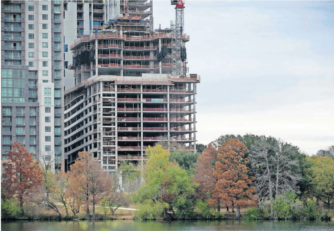
The 44 East Ave. project is under construction in Austin. The tower is adding to the ongoing growth boom in the Rainey Street District, which is along downtown Austin's southeastern edge. [JAY JANNER/AUSTIN AMERICAN-STATESMAN]
